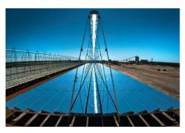
Areva's solar unit consisted of what remained of the acquired startup Ausra and its compact linear Fresnel reflector (CLFR) solar steam generator technology.
